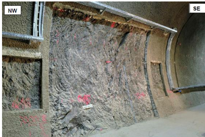
Mont Terri: exposed fracture network.
