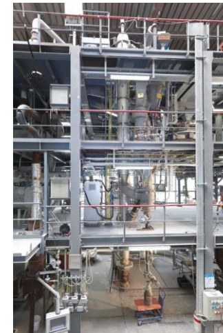
Pilot-scale calciner and 4 stage pre-heater - tkIS
